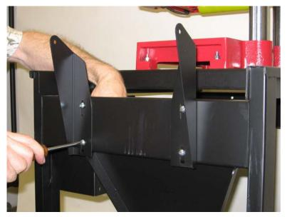
Mount the vertical roller support brackets in pairs, left and right hand on both ends of the stand. Use 1/4"x 5/8" long round head screws, lock washers and nuts.
